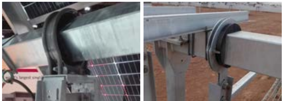
Image 11 y 12: Example of a commercial cylindrical bearing
