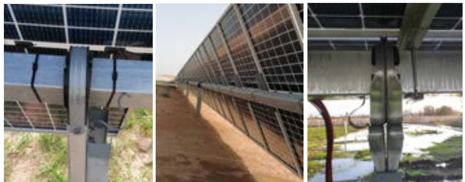
Images 37, 38 & 39: Spherical bearing assembling example
