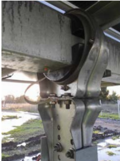
Image 6: Spherical bearing assembled in Vanguard 2P
