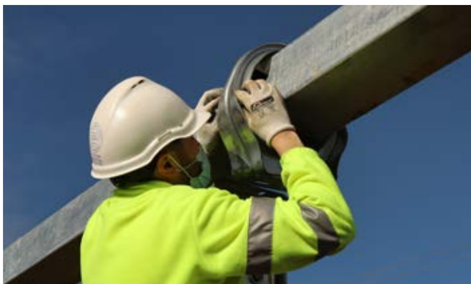
Image 5: Spherical bearing installed in Habei, China, 400 MW
