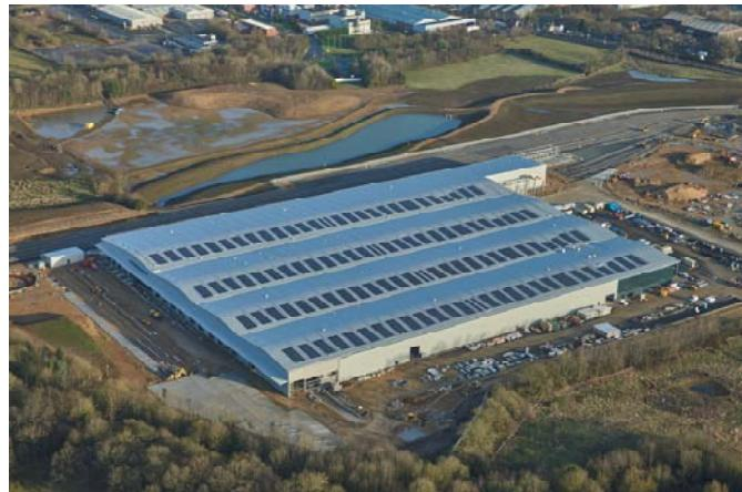
Photon Energy to complete the commercial rooftop installation at the Hitachi Rail site in Newton Aycliffe where 3,772 Honey M 265W modules were deployed. Initially, the project was specified to be completed with 250W modules; however with the decision to install Trina Solar's higher performing monocrystalline Honey M 265W modules, it was calculated that a substantial Balance of System (BOS) saving of 100kW could be made, making the installation economically viable.
