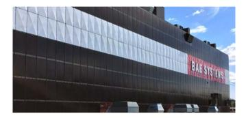
The completed project has enabled BAE Systems Hägglunds to make pioneering changes to the way it powers its facilities, as well as improve its external appearance. With a projected annual energy output of 312 MWh, fully consumed on site, the new installation is set to significantly reduce the company's reliance on non-renewable energy sources.
